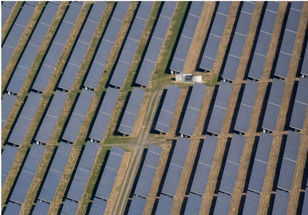
Rows of solar panels.
